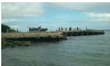
UPGRADING OF AZAGRA FEEDER PORT PROJECT, ROMBLON
