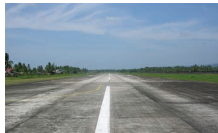
ORMOC AIRPORT PROJECT, LEYTE
