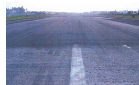
KALIBO AIRPORT DEVELOPMENT PROJECT, AKLAN
